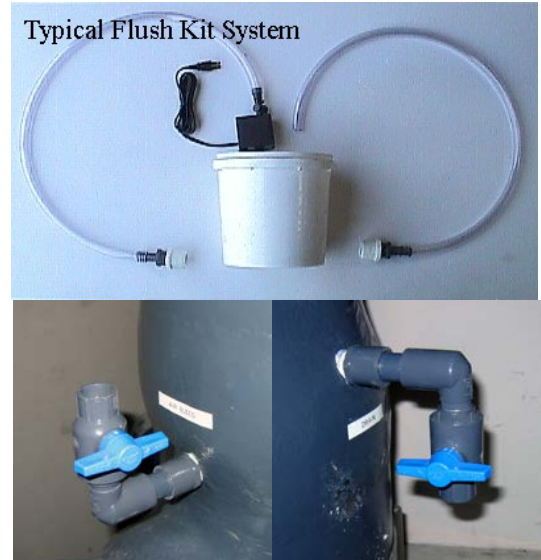
Air Bleed and Drain Valves
